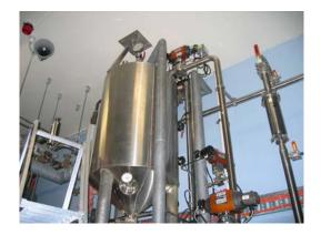
**Description**: This boiler is mounted too high, with a burst disk near the top. **Pitfalls**: When the boiler is mounted too high, it is extremely difficult to service. Lag spots are present, and temperature probe testing reveals poor circulation. **Suggested precaution**: Mount boilers where they will be easy to monitor and service.
