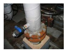
**Description**: Room humidity and cool air temperature causes condensation of water on non-stainless-steel pipes, causing rust.
