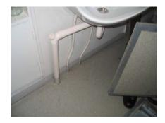
**Description**: Unsealed floor without coving. **Pitfalls**: Visible holes reveal non-waterproof outlets that are not airtight, preventing hosing down. Improperly sealed retrofitting is another common problem. **Suggested precaution**: Properly seal walls, floors, and equipment. Extend floor covering at least six inches up the walls (coving).
