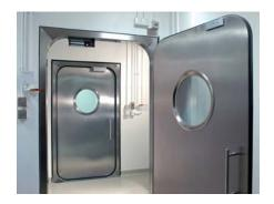
**Description**: This large airlock at the University of Hong Kong features air inflatable door seals that are flush with the floor.
